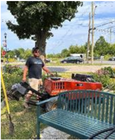
Installation of the watering system
